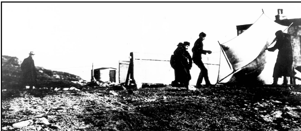
Marconi and helpers at St. John’s, Newfoundland launching a kite to support a long receiving aerial wire in December, 1901.
